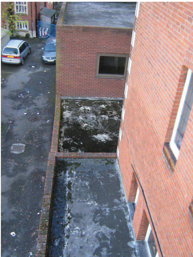
Photo 6. Flat roof over the staff entrance
