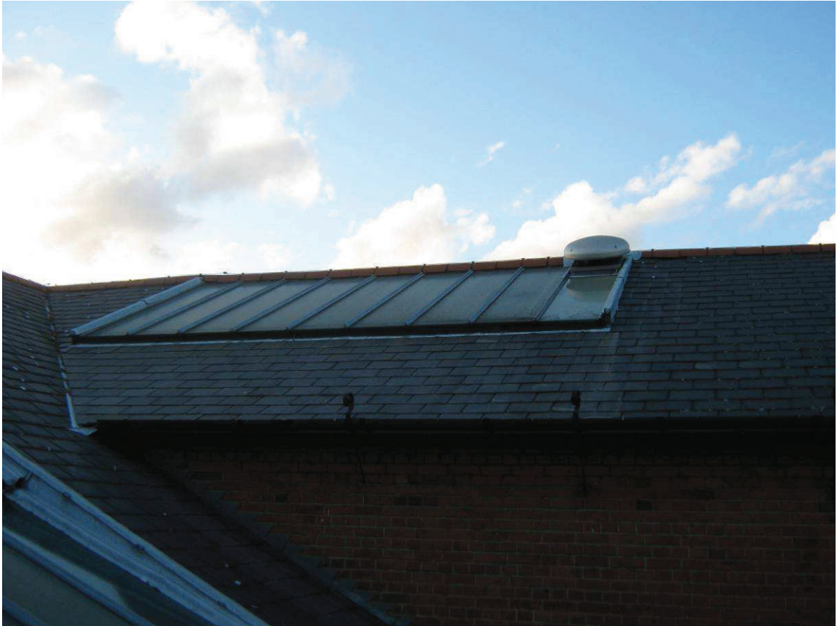
Photo 3. Roof light over reference library
